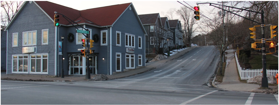
Bedford Highway at Meadowbrook Drive looking west
