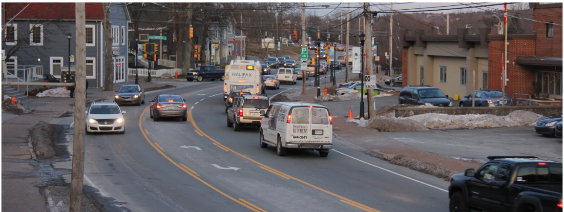
Bedford Highway approaching Meadowbrook Drive to the north
