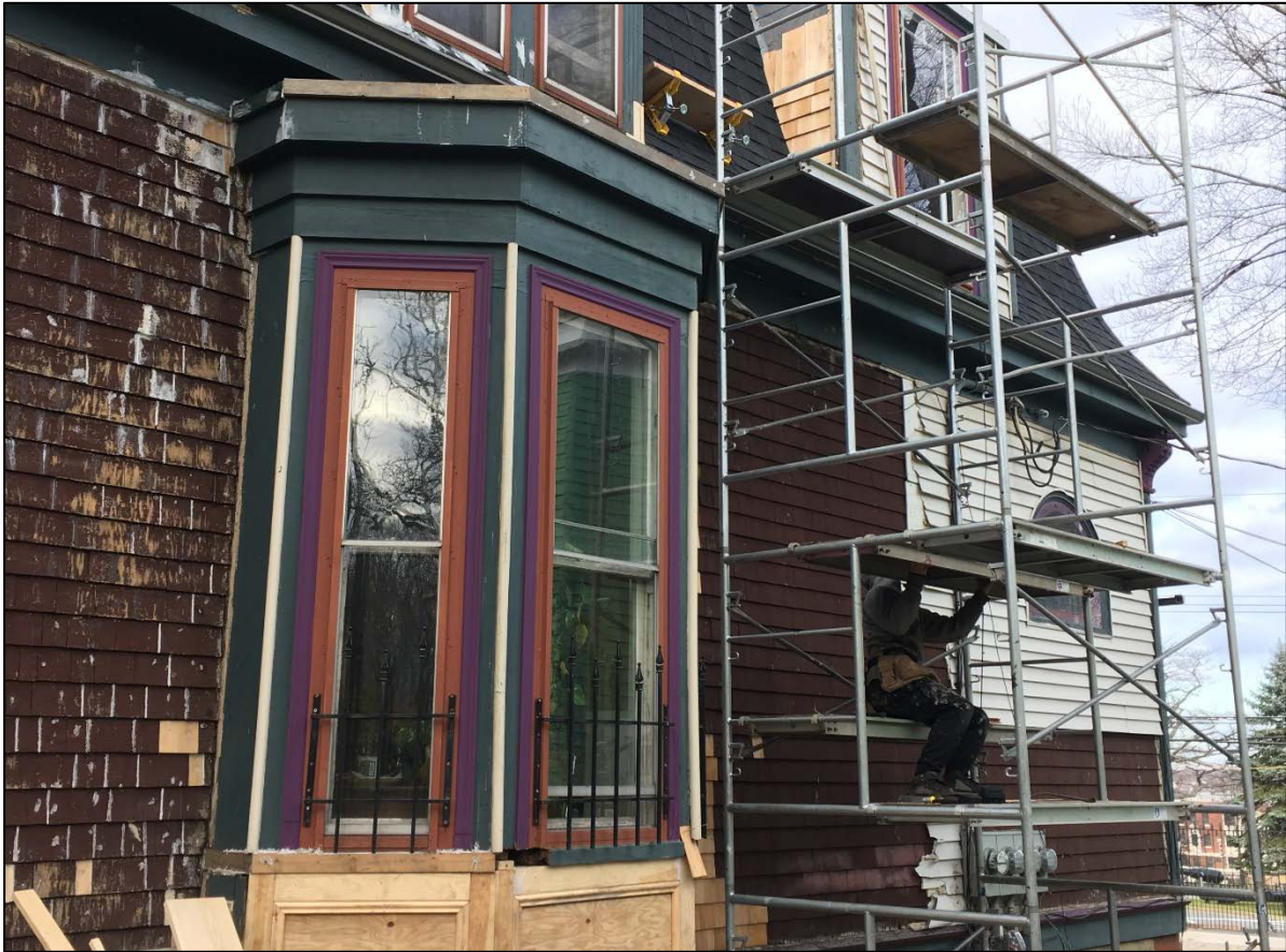
Exterior Restoration (Removal of Vinyl Siding and window conservation).
