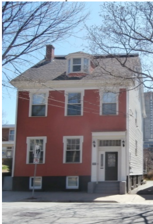
Detached “Halifax House” on Morris Street with truncated gable roof and Scottish dormer
