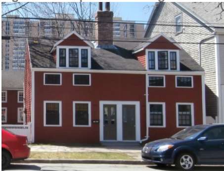
One-and-a-half storey mirror image houses with shared gable roof and prominent brick chimney
