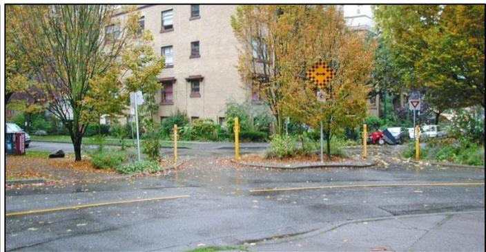
Figure 7: Photo of Diagonal Diverter in Victoria BC
