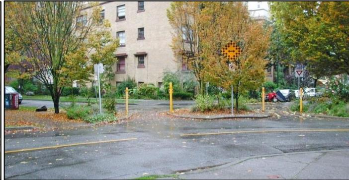
Figure 5: Photo of Diagonal Diverter in Victoria BC
