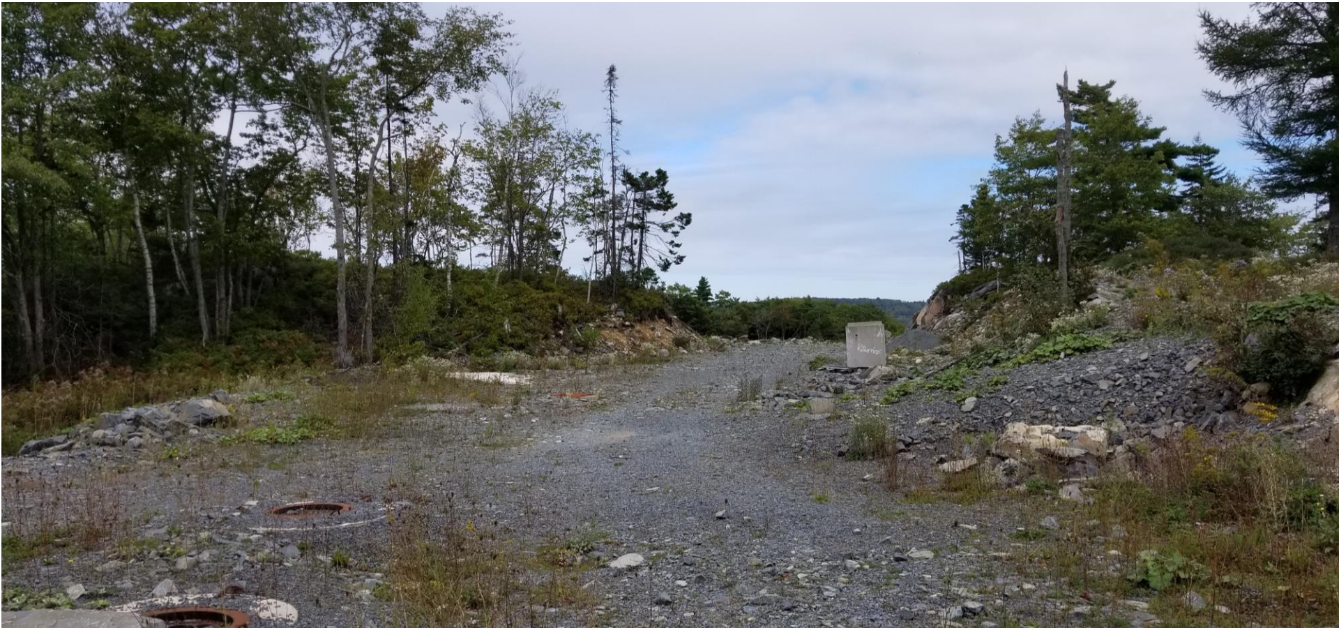
Site entrance off Larry Uteck Blvd.
