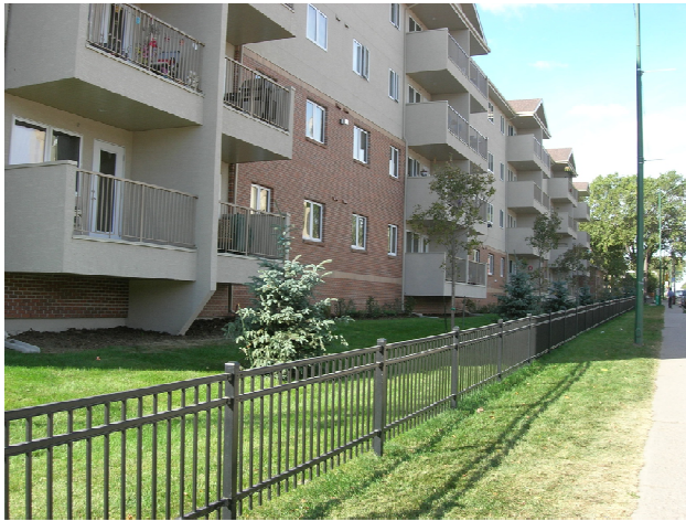
The Province provided funding to KC Charities Inc. to build this 75 unit affordable housing project for seniors in Pleasant Hill Village.
