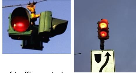
Commonly called flashers or flashing lights, these are a type of traffic control signal that continually flashes amber or red at intersections or in advance of a location which would require the driver to take greater care due to unusual conditions.
