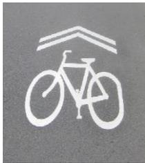
A shared use lane marking or “Sharrow” is a pavement marking indicating to motorists and cyclists that a lane is to be shared by vehicles and bicycles. The marking designates the preferred positioning in the lane for cyclists and may be located for single file movements or side by side, shared with motor vehicles.
