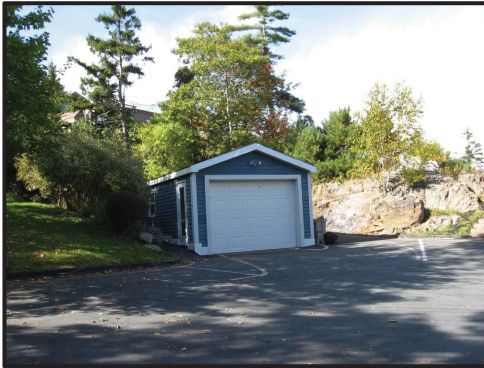
Garage on Lot G1 (upper portion)
