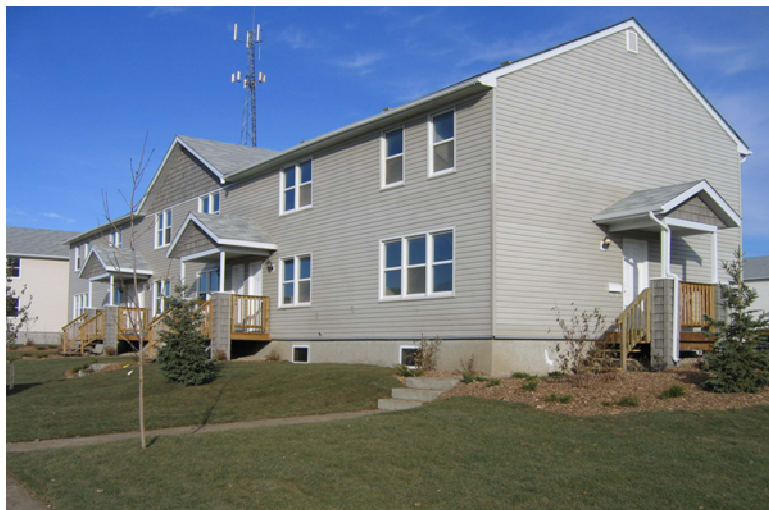
Affordable ownership housing. These completely renovated units were re-located from McNab Park to Camponi Place.
