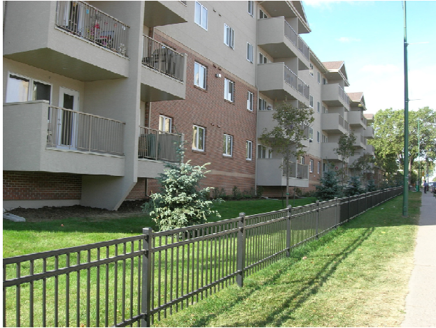
The Province provided funding to KC Charities Inc. to build this 75 unit affordable housing project for seniors in Pleasant Hill Village.
