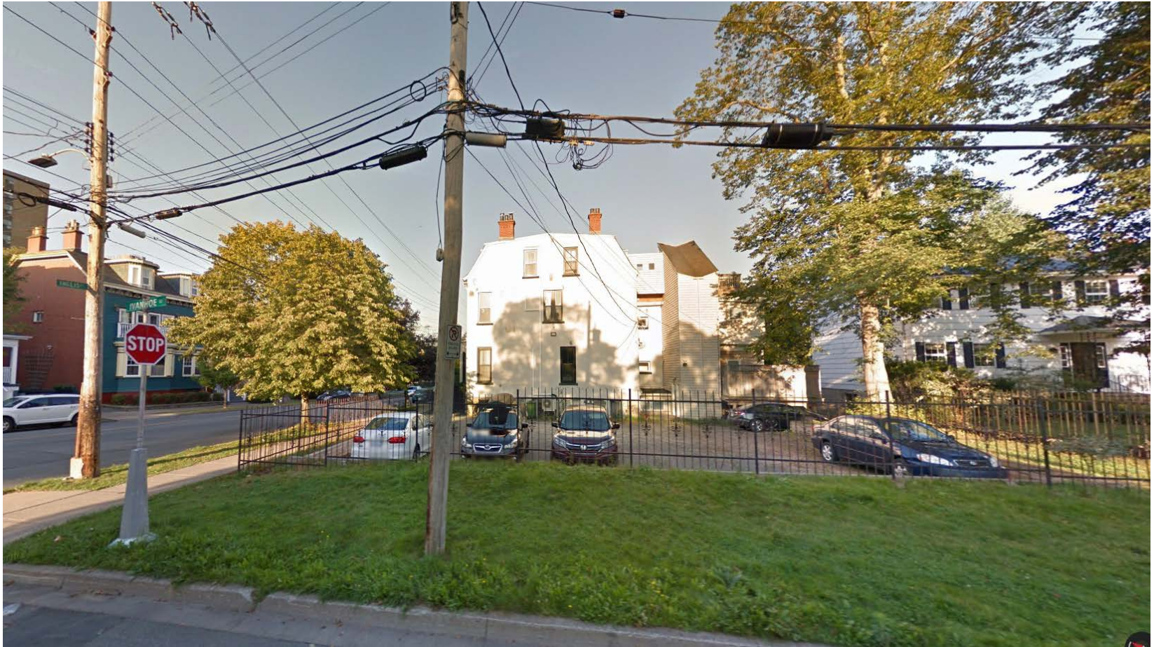
Subject Property from Ivanhoe Street
