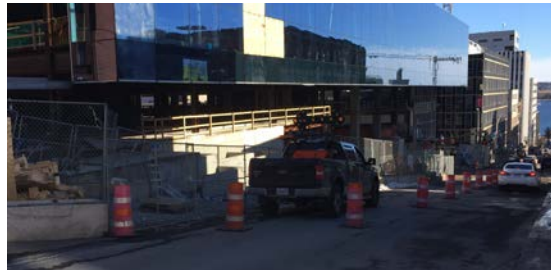
Figure 2 – Traffic Control in a dense urban environment.
