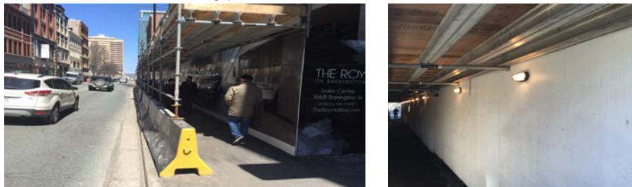
Figure 5 – Solid construction hoarding provides pedestrian protection from vehicles, overhead objects, and provides physical separation from the site activities. Lighting for covered ways is an important consideration.
