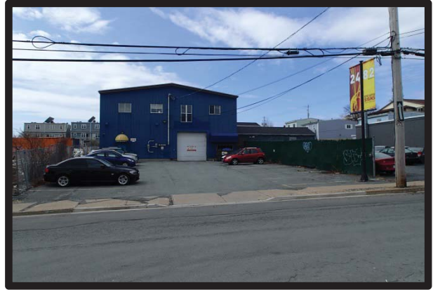
Sign fabricator shop immediately to the north of the subject site, along Maynard Street
