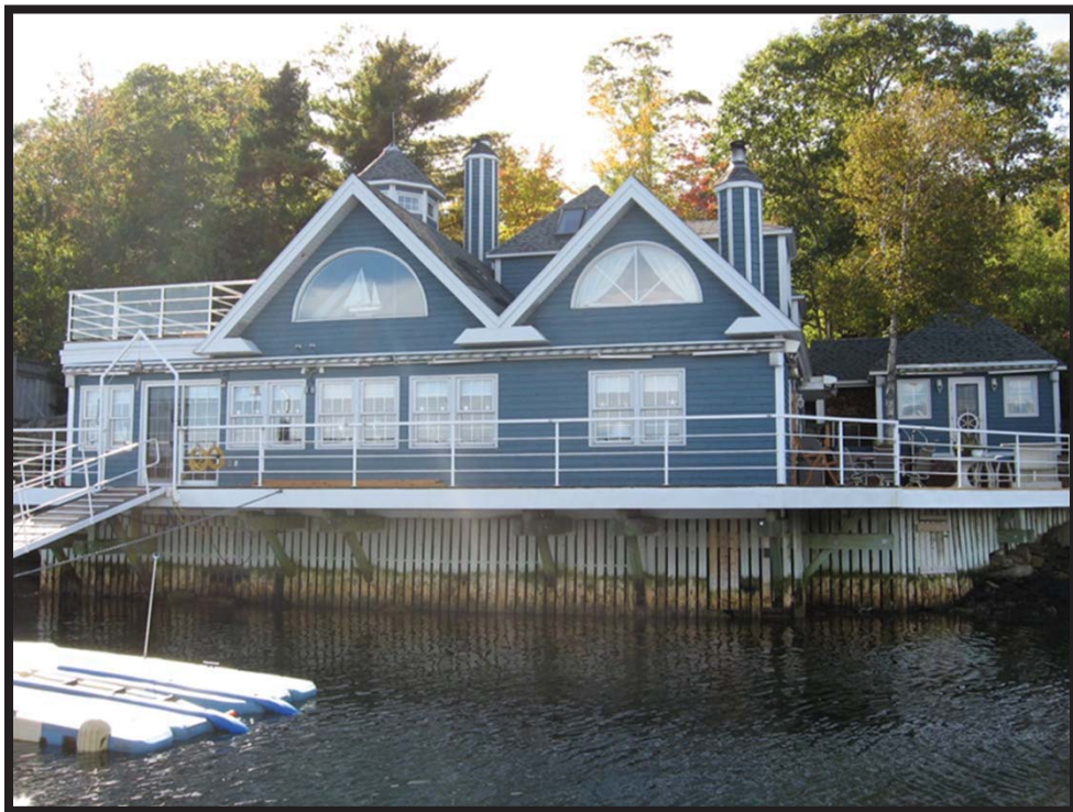
Dwelling on Lot G2 (from dock)
