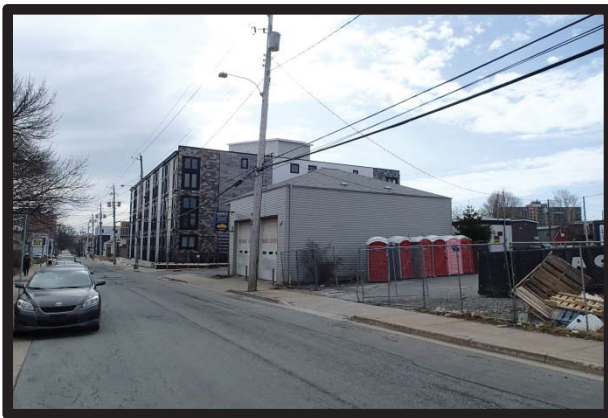
Q Lofts Building, with 2740 Maynard and subject site in foreground
