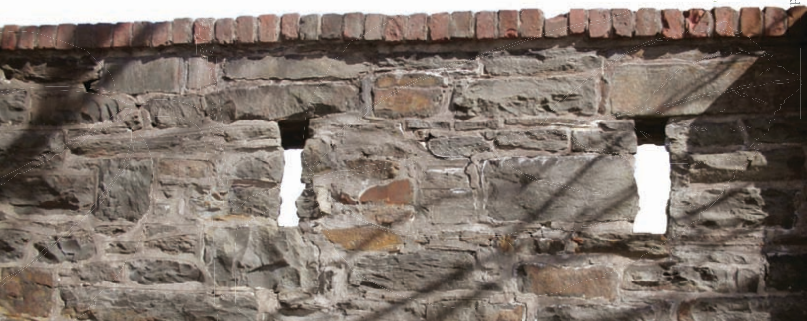
Perimeter wall at Fort Ogilvie
