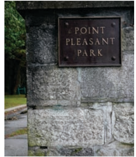
Tower Road gate
