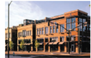
Figure 12. Retail and commercial uses conceal the parking structure from the streetscape
