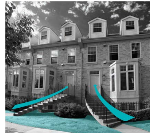
Figure 44. Individually accessed residential units with a landscaped front yard setback and raised entrances respond to surrounding neighbourhood form.
