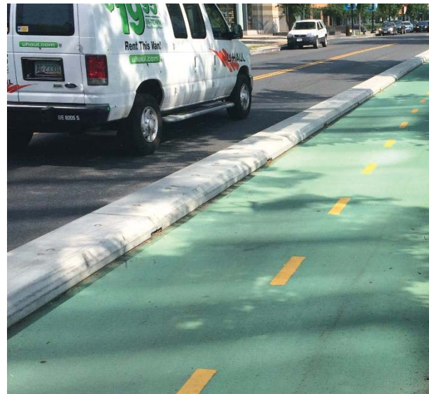
Figure 7: Example of low-profile pre-cast concrete curb (Washington, DC; source: M. Connors)
