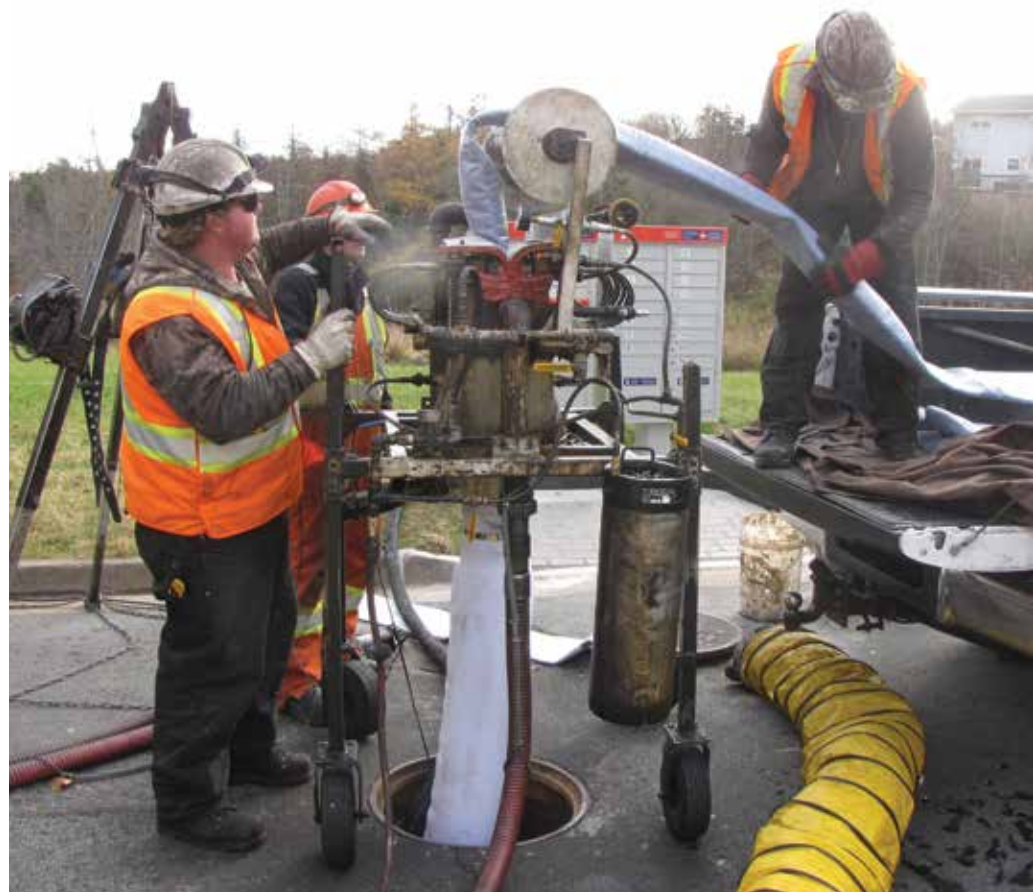
Sliplining a wastewater pipe to reduce inflow & infiltration
