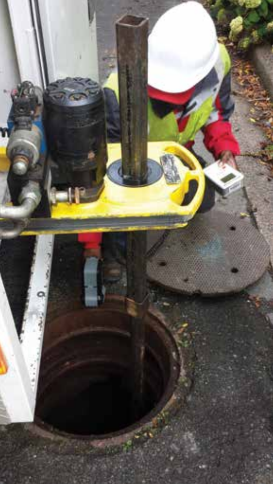
Field Crews Rehabilitated Critical Large Water Valves on the Halifax Peninsula
