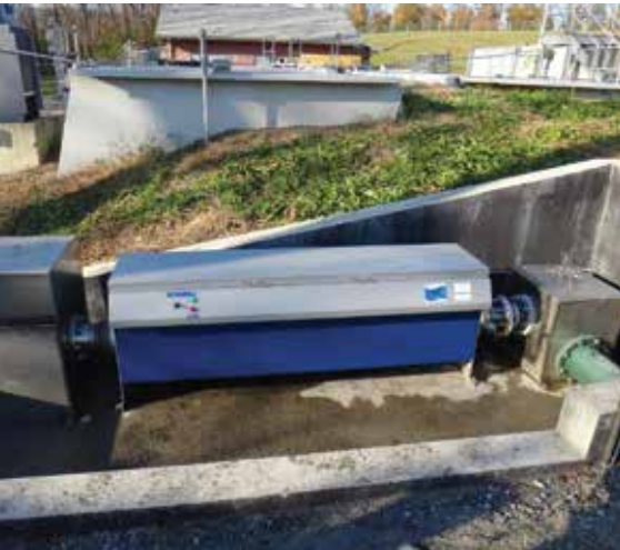
Example of UV system to be installed at the Springfield Lake WWTF
