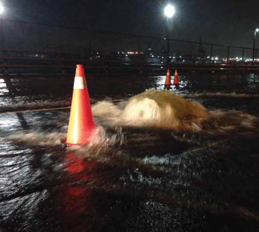
Overflowing manhole discharges into the street during a significant rain event
