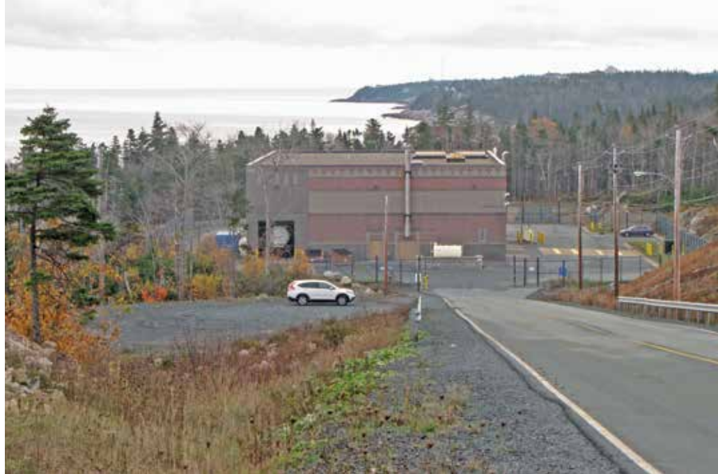
Herring Cove WWTF, a tranquil setting in the Outer Harbour
