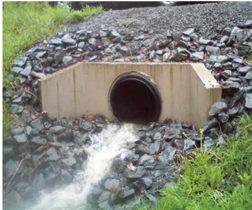
Culvert Inventory & Condition Assessment Completed by Asset Management Team
