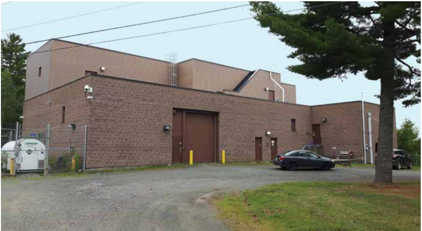
Bennery Lake Water Supply plant
