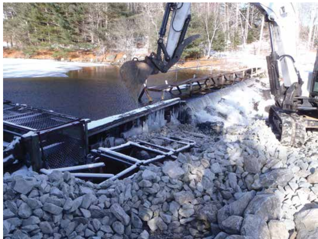
Stabilizing the fish ladder at the Lake Major dam January 17, 2015
