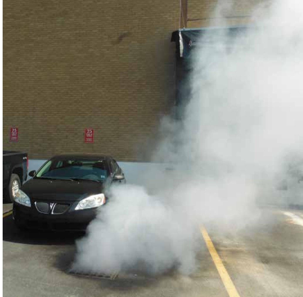
Right: Environmental Engineering staff use smoke testing to find stormwater connections to the wastewater system
