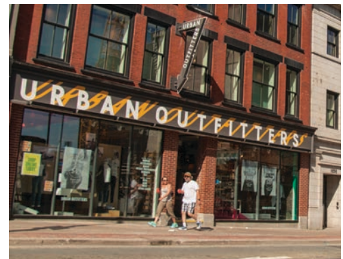
Figure 84. Fascia signs shall be located in the architectural frieze above the storefront.
