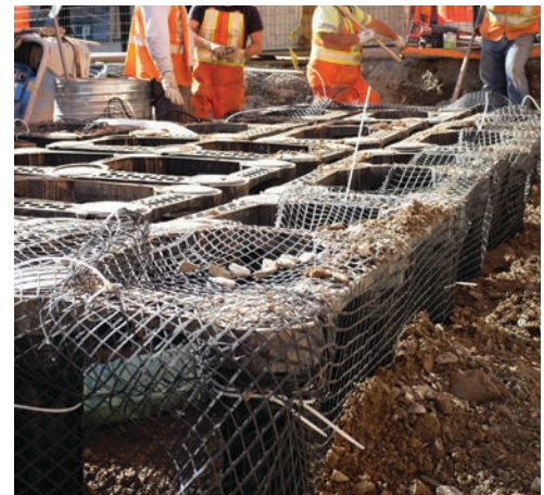
Figure 30. Silva cell technology minimizes subsurface compaction, enabling stormwater conveyance and healthier tree rooting systems
