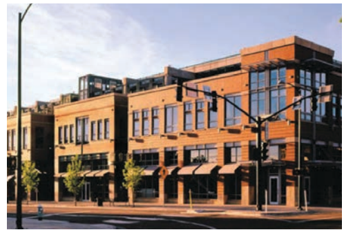
Figure 12. Retail and commercial uses conceal the parking structure from the streetscape
