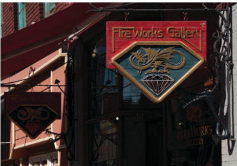
Figure 86. Locate projecting signs that identify a ground floor business above or adjacent to the entrance to the business premises.
