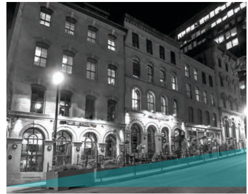
Figure 20. Active frontage with spill-out activity along a slope.
