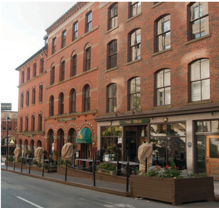
Figure 57. The fenestration shapes and pattern are defining features of the building.
