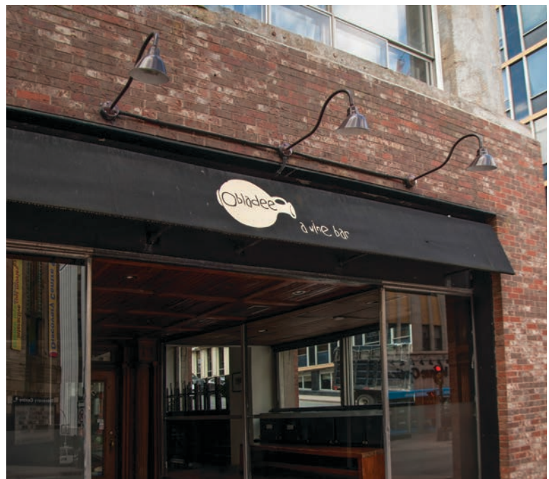
Figure 77. Awning is designed to fit within the dominant horizontal structural elements of the lower façade.
