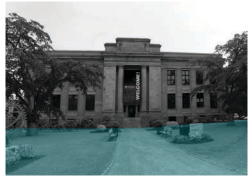
Figure 7. Emphasize prominent View Terminus sites and prominent civic frontages through the strategic siting of buildings and open spaces
