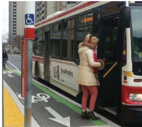
Figure 13: Shared cycle track-bus stop on Roncesvalles Avenue, Toronto (Source: MTO Book 18)
