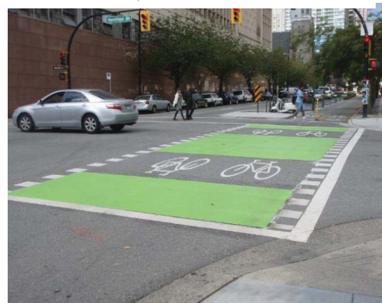
Figure 9: Intersection crossing markings on bi-directional bikeway in Vancouver (Source: Alexander Pope, flickr.com; creative commons license)
