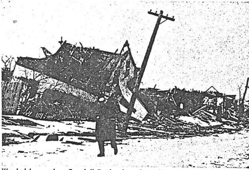
Wrecked houses along Campbell Road, a busy thoroughfare near the waterfront in the Richmond section of Halifax. In the town of Sydney, 200 miles to the north, people sitting down to breakfast saw their plates move
