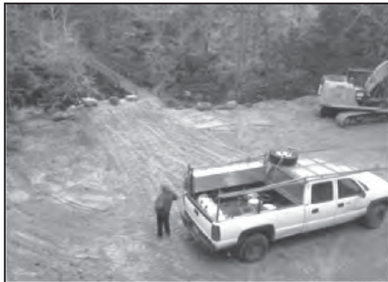
The area where the new bridge will be installed.
