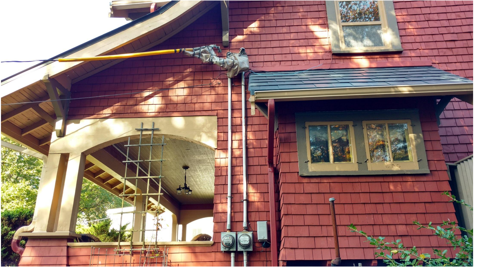
Figure 6: South facade showing front porch supported by columns set on low pedestals sheathed with wooden shingles
