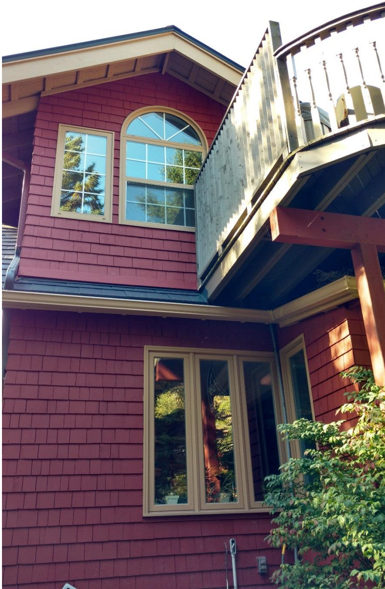
Figure 9: East facade with rear addition and deck
