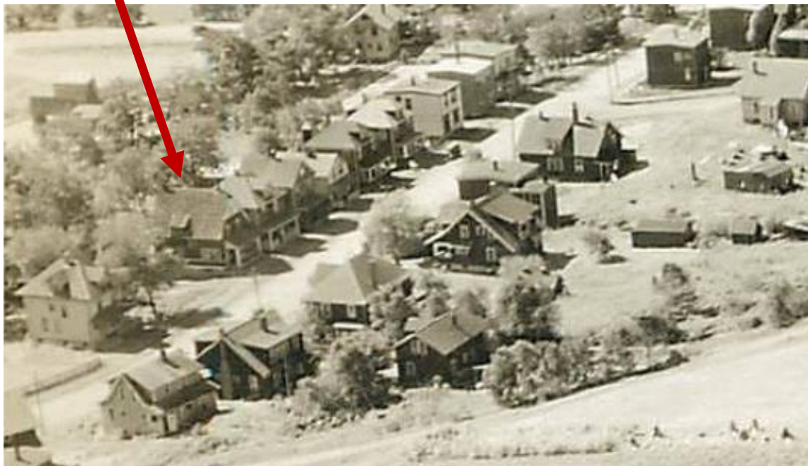
Figure 2: Aerial photograph taken in 1929 (Dunn, Ross)
