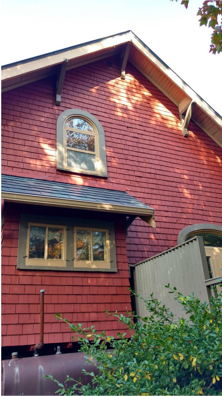
Figure 7: South facade continued showing large ornamental brackets
