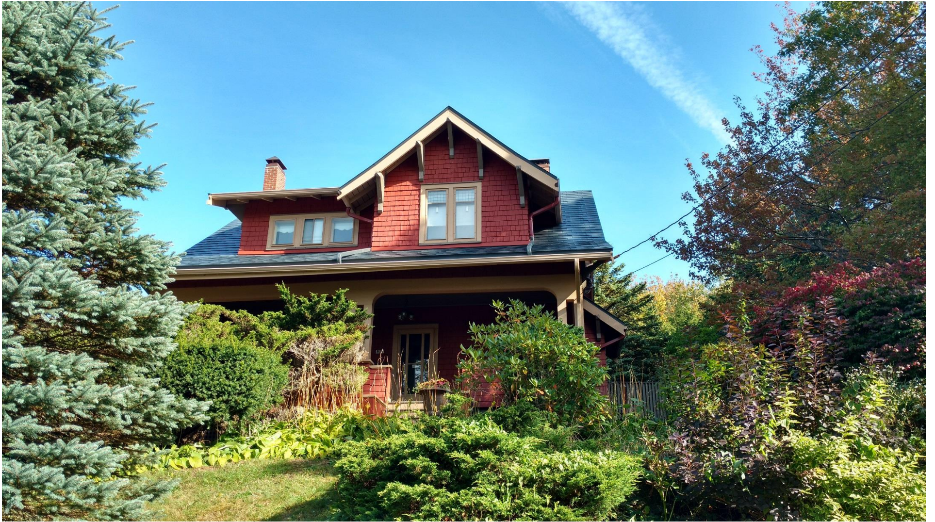
Figure 1: West Elevation (facing Hawthorne Street)
