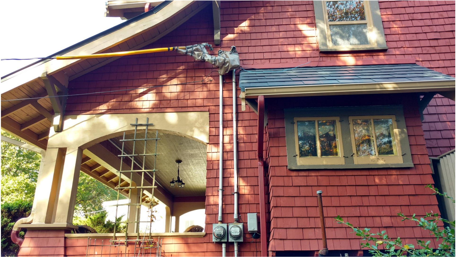
Figure 6: South facade showing front porch supported by columns set on low pedestals sheathed with wooden shingles
