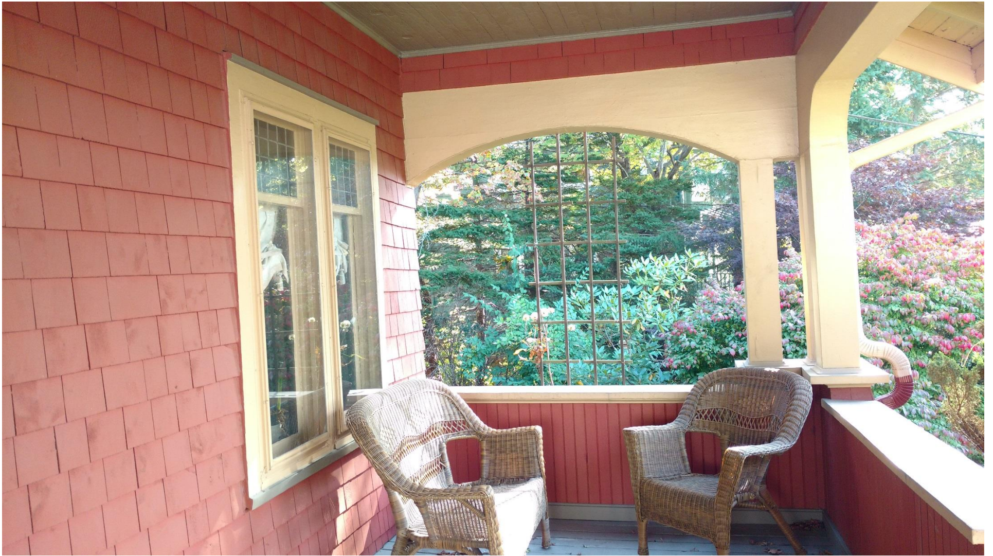
Figure 5: Front porch framed by arched beams and double-hung, multi-pane windows with wide casings
