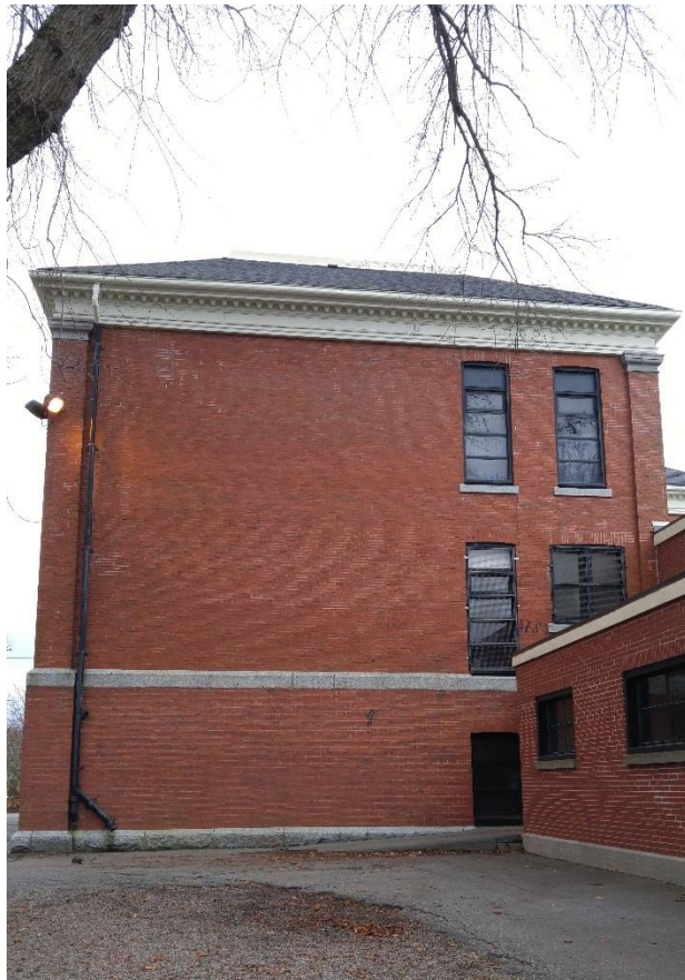
Figure 6: East elevation showing rear of heritage building
