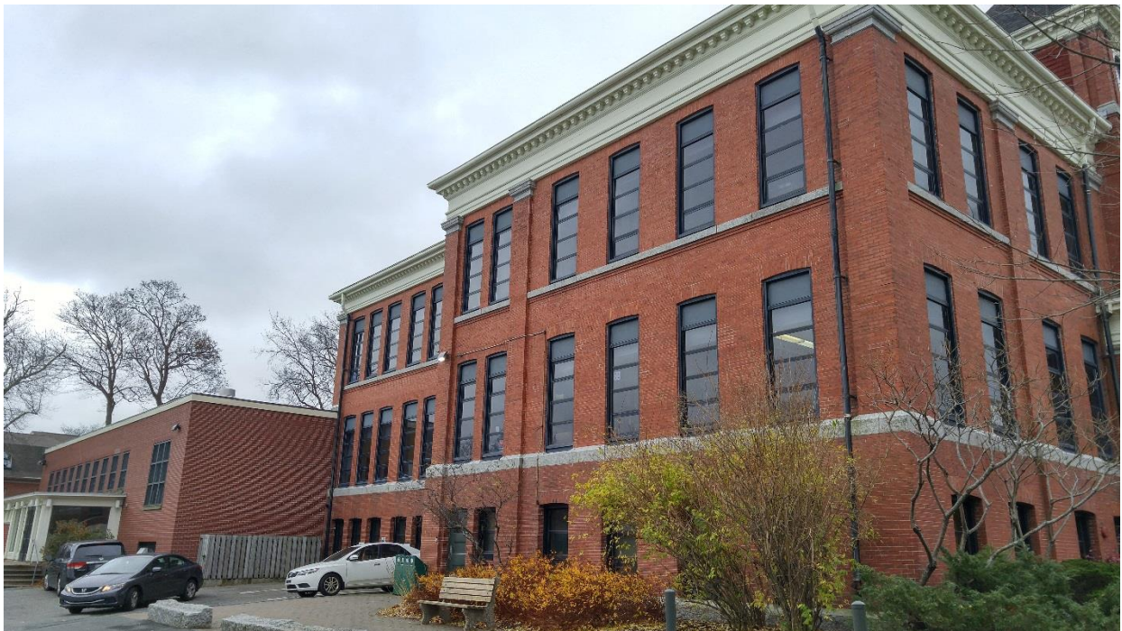
Figure 2: North elevation showing heritage building and 1950s addition
