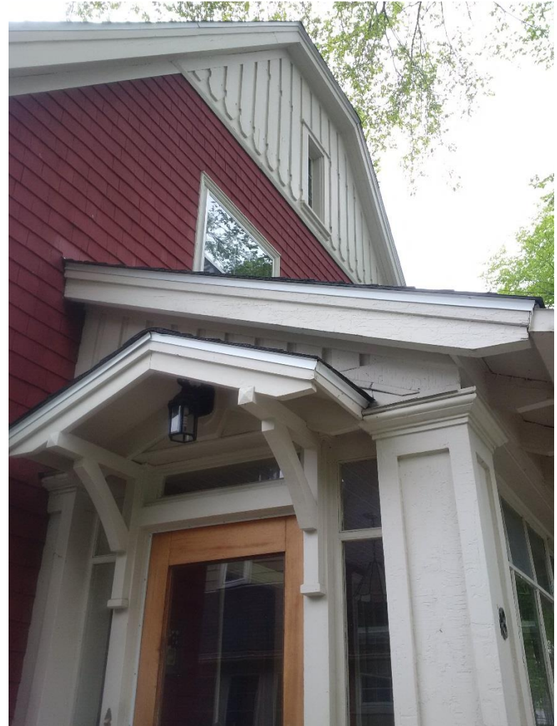
Figure 6: Enclosed porch with side entrance
