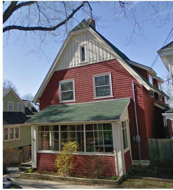
Figure 9: Front elevation of subject property
