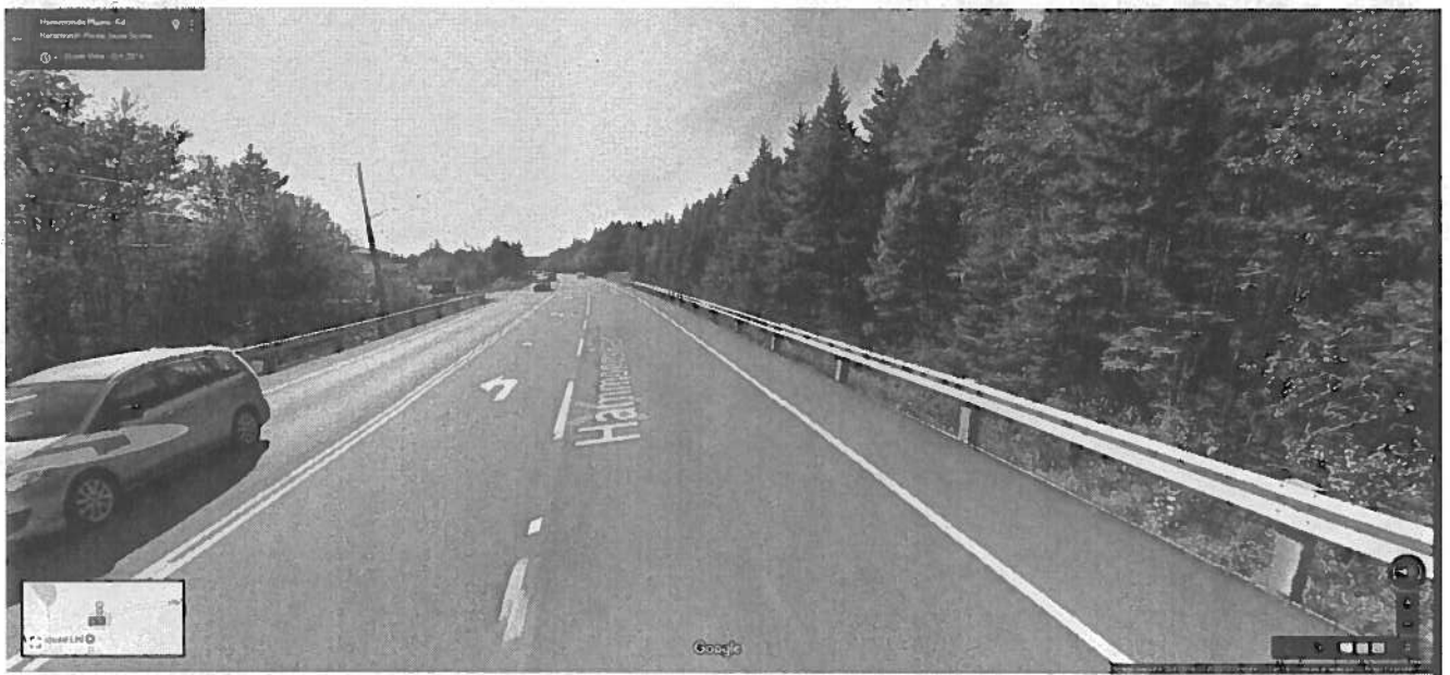
Intersection of Hammonds Plains Road and Yankeetown Road, October 2016
