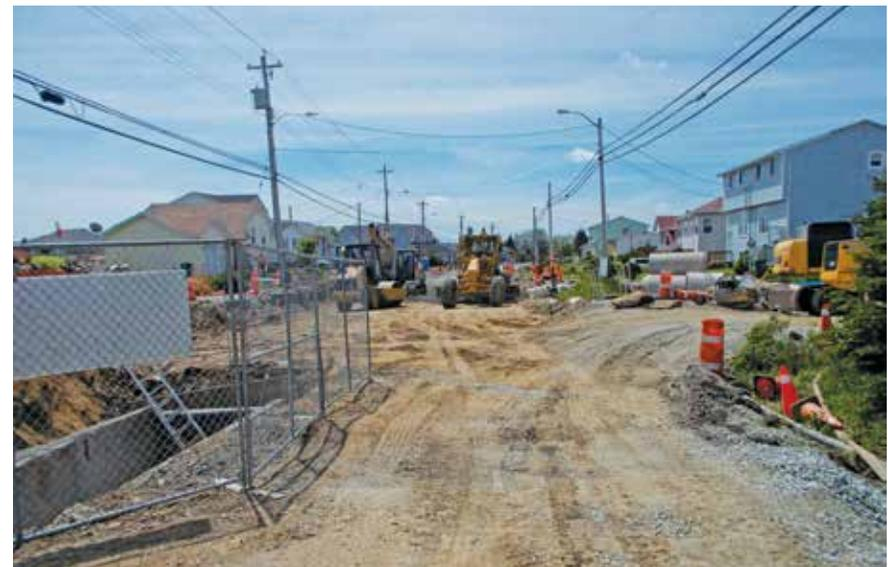
**Cow Bay Road deep storm sewer project—getting stormwater out of the wastewater system**
