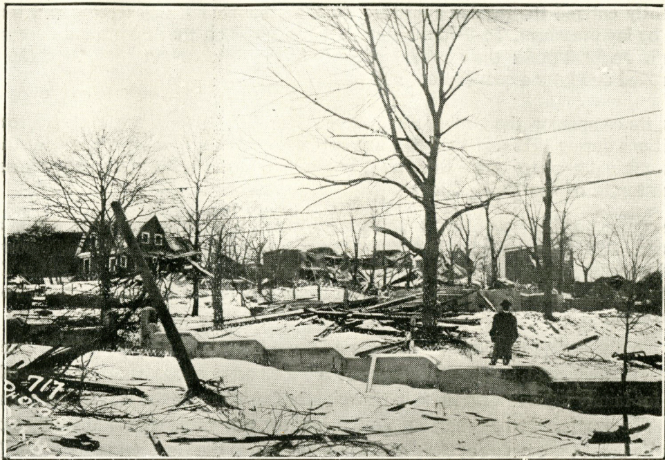
KAYE STREET METHODIST CHURCH RUINS AFTER THE DISASTER
