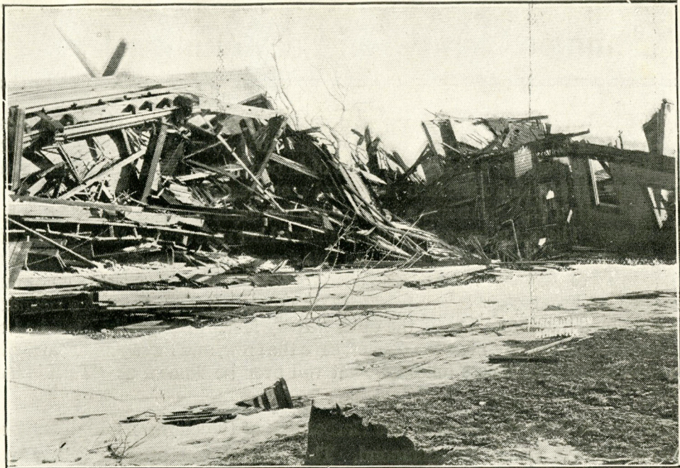
GROVE PRESBYTERIAN CHURCH AND HALL AFTER THE DISASTER
