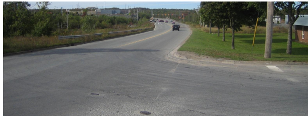
Photo 5 - Looking north on Duke Street towards Damascus Road and Highway 102 from the Mann Street intersection.
