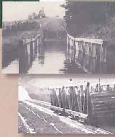
An empty cradle car sits in the water at the bottom of the inclined plane.
