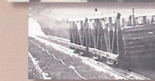
A cradle car and canal boat on its way up the inclined plane.
