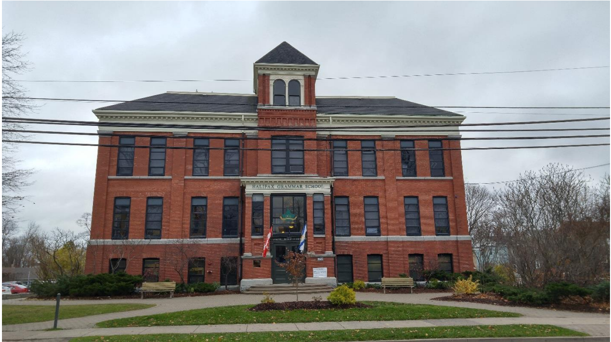
Figure 1: West elevation showing front entrance to existing school
