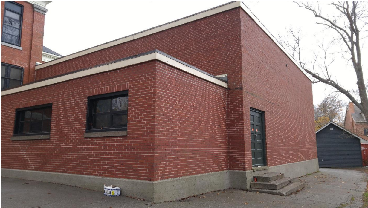
Figure 5: East and south elevation showing 1950s addition
