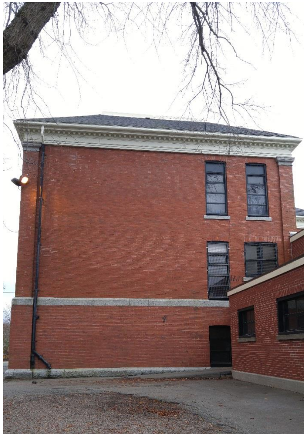
Figure 6: East elevation showing rear of heritage building
