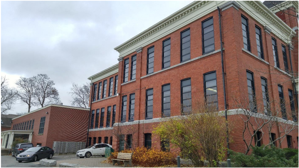
Figure 2: North elevation showing heritage building and 1950s addition
