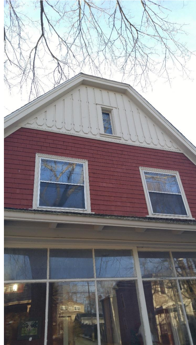
Figure 2: Decorative vertical boards or sticks with fixed window below hipped gable and two evenly placed eight-over-one hung windows
