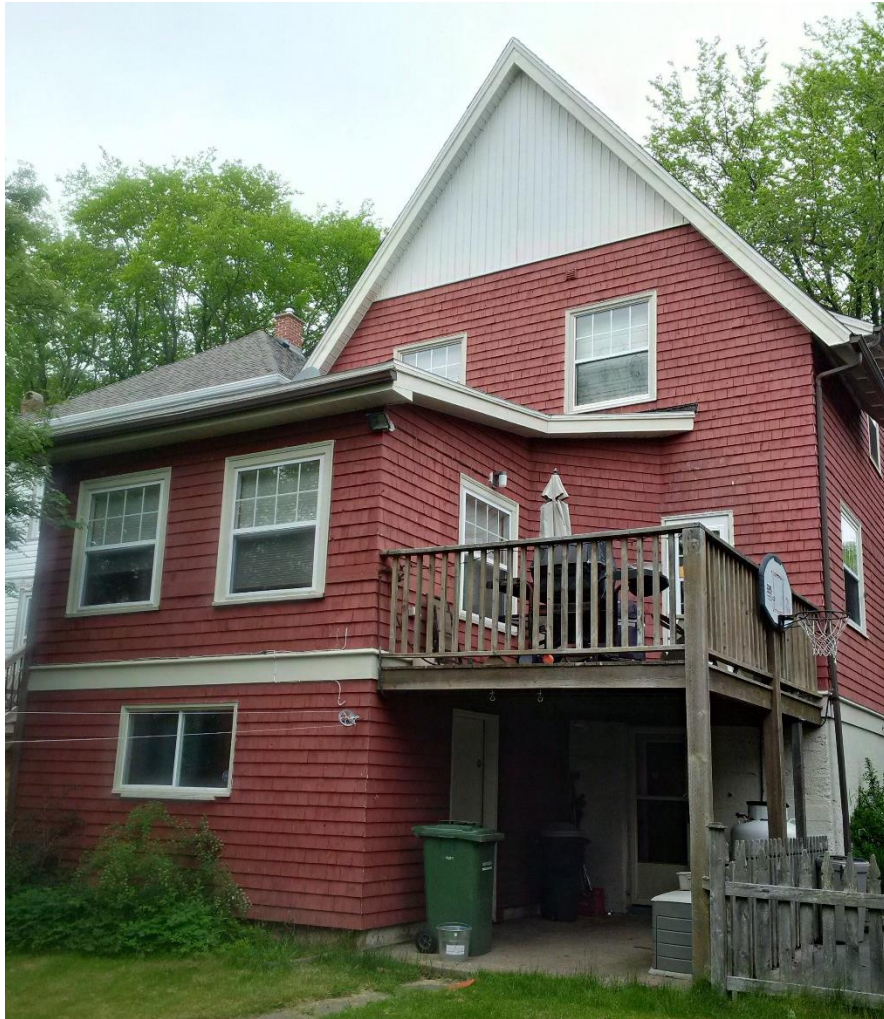
Figure 5: South or rear elevation showing 1980s addition and deck
