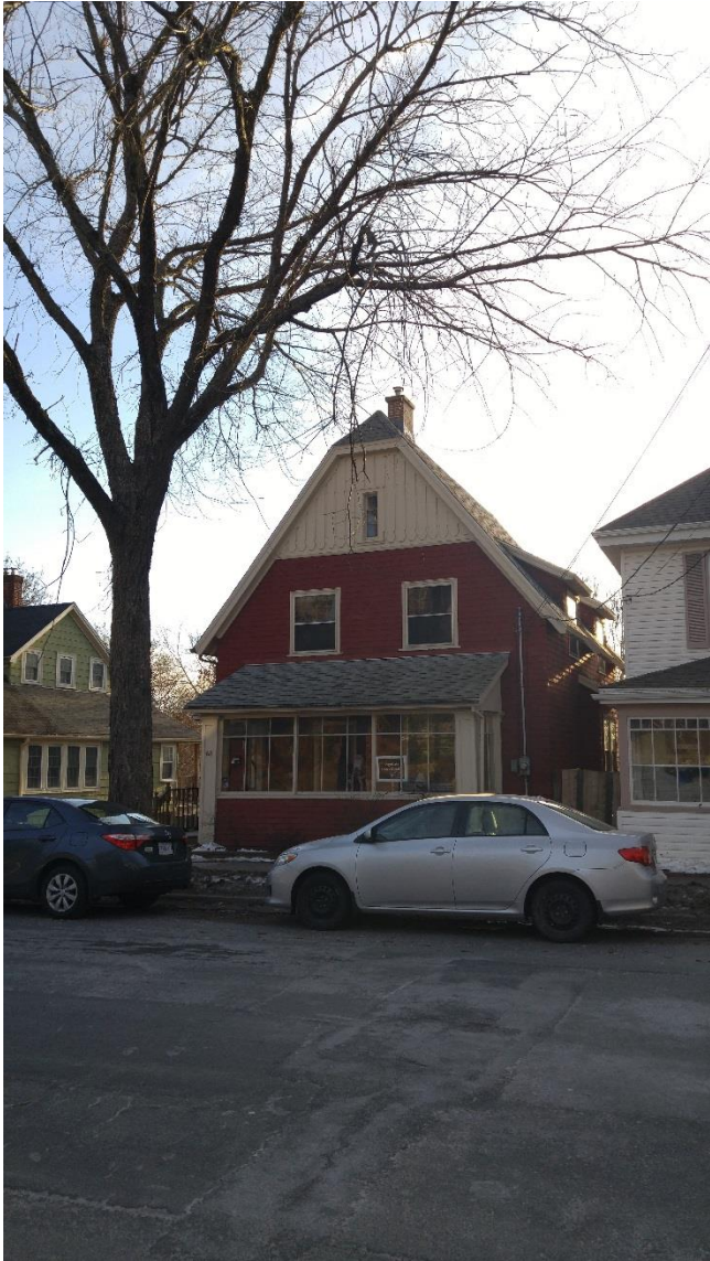
Figure 1: Front elevation steep pitched gable roof with hipped gable, and front porch
