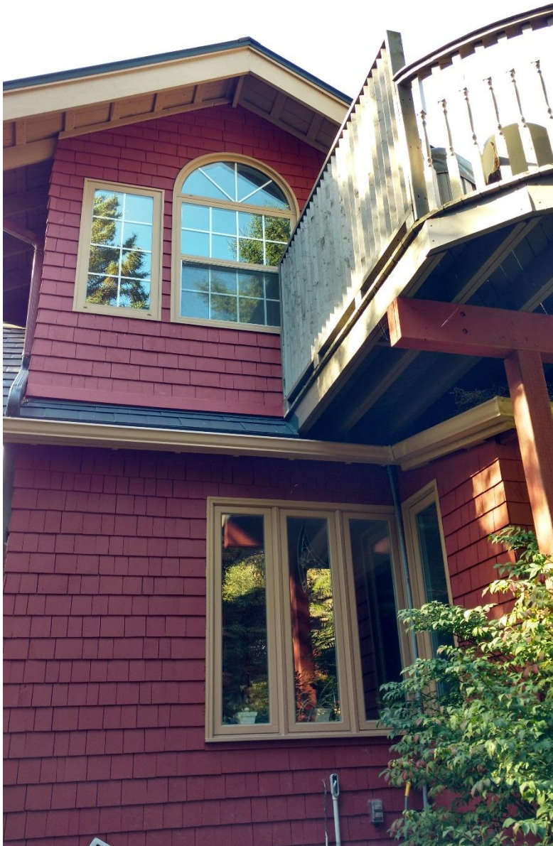
Figure 9: East facade with rear addition and deck
