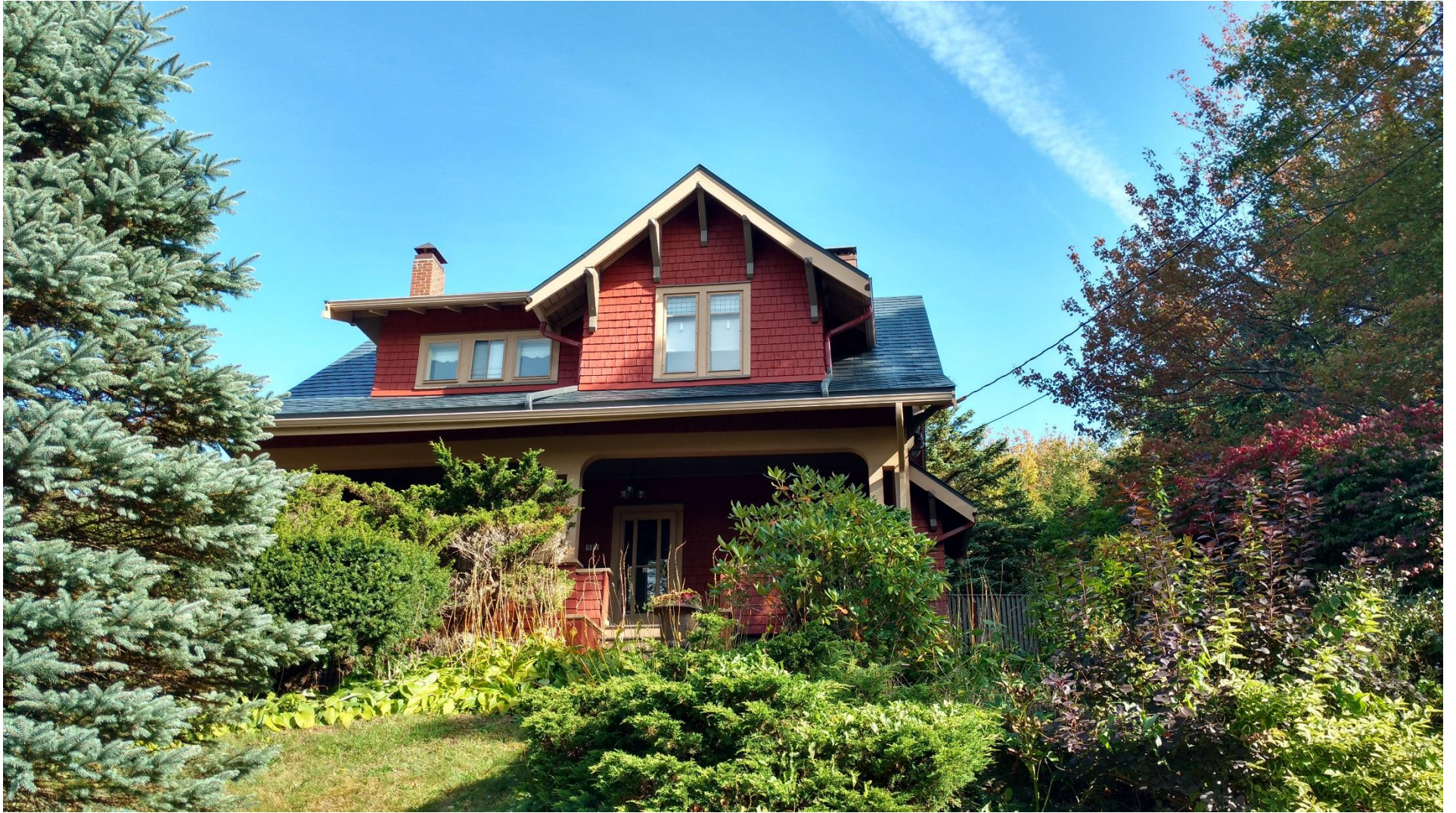
Figure 1: West Elevation (facing Hawthorne Street)
