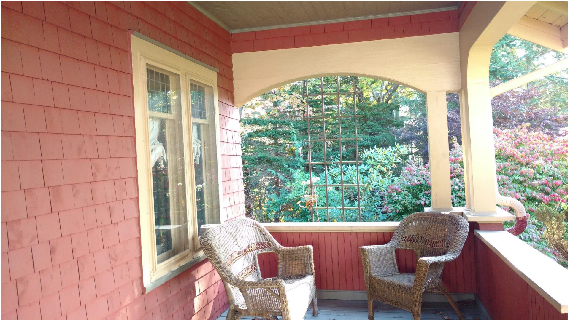
Figure 5: Front porch framed by arched beams and double-hung, multi-pane windows with wide casings
