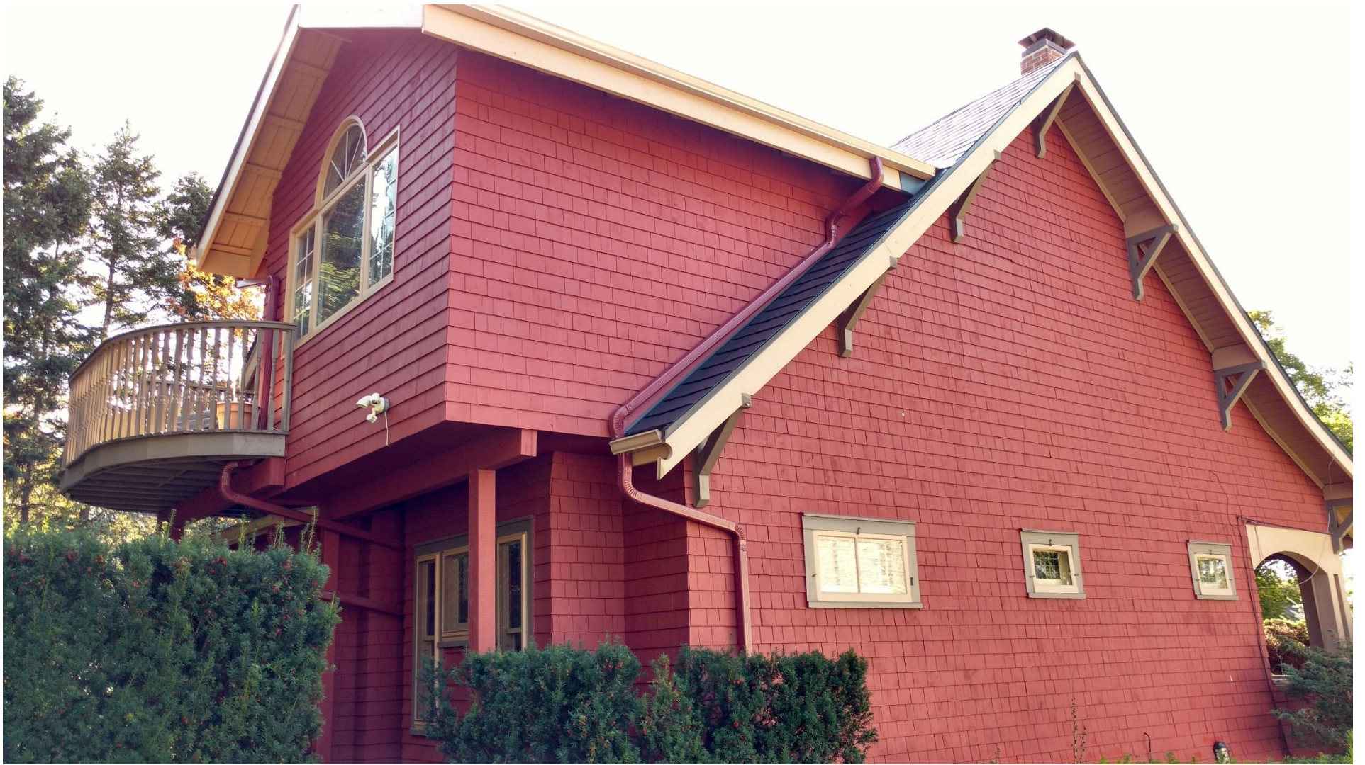
Figure 11: North facade showing rear addition, medium pitched gable roof with large decorative brackets under gable eaves, and piano windows
