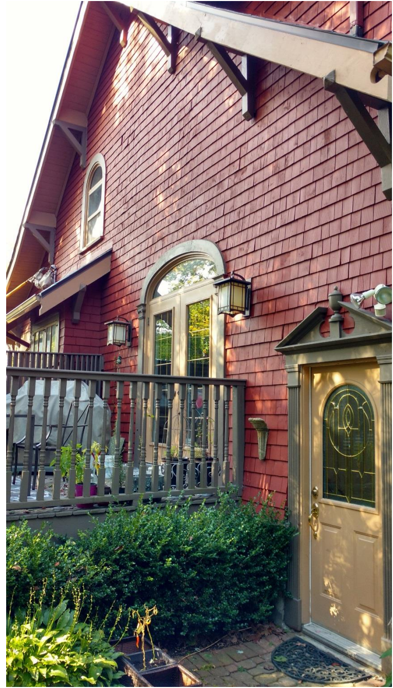
Figure 8: South facade continue
