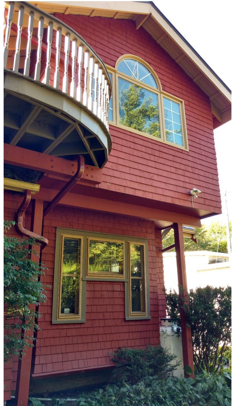
Figure 10: East facade continued
