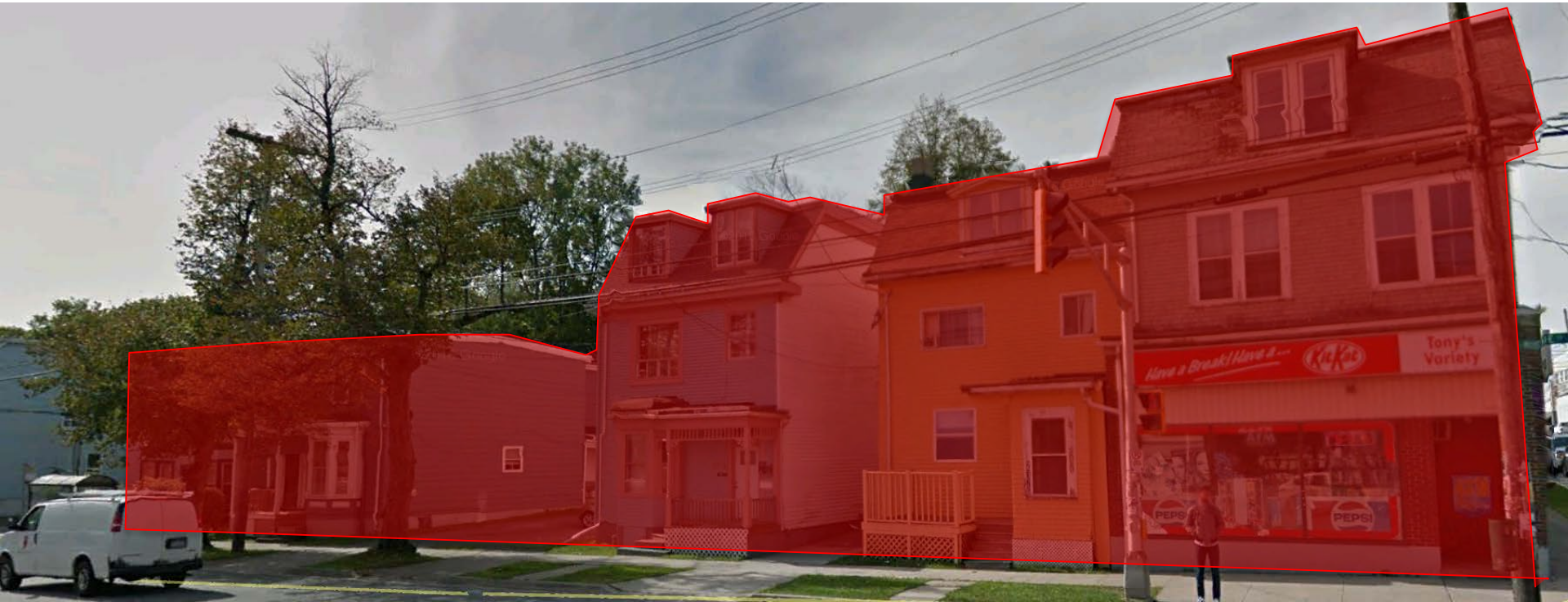
Subject site seen from the northwest, corner of Robie Street and Cunard Street
