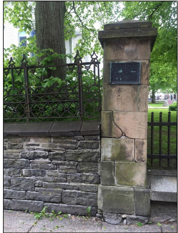
Figure 2: Sandstone pillar on Barrington Street.
