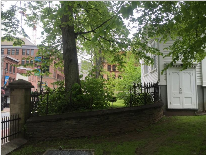
Figure 1: Wall section on Barrington Street abutting the Church.
