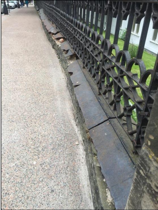
Figure 12: Bowed wall section & broken metal wall cap.
