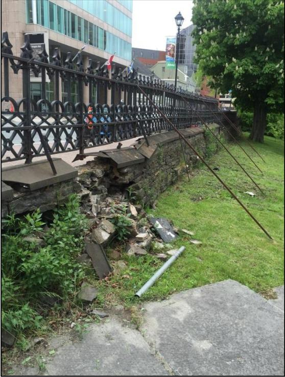
Figure 11: Failed wall section on Argyle Street.
