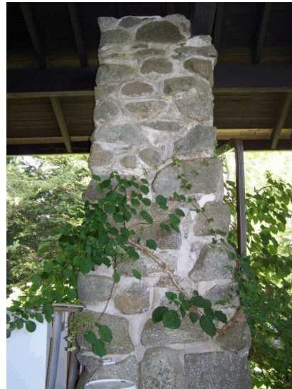
Main house - porch column.
