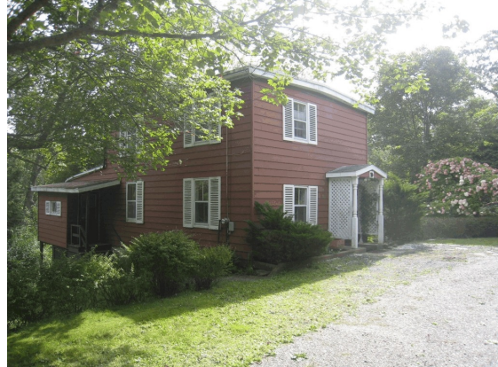
The Gate House, 2009.
