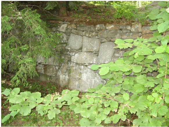
5' high dry stone wall (near main house).
