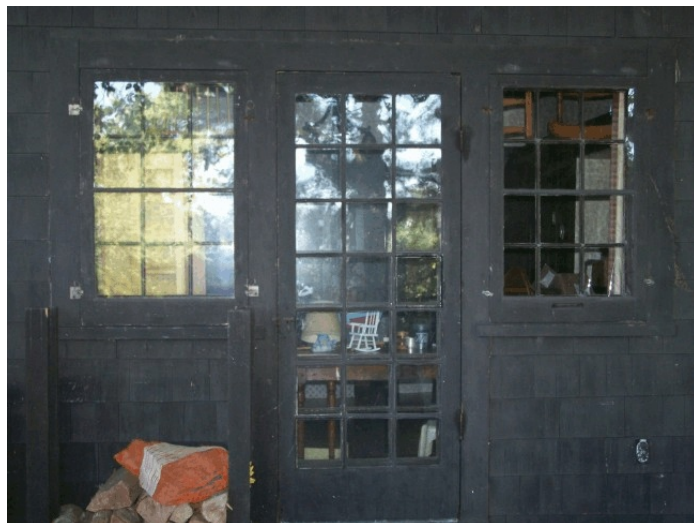
Main house - secondary entrance on front elevation.
