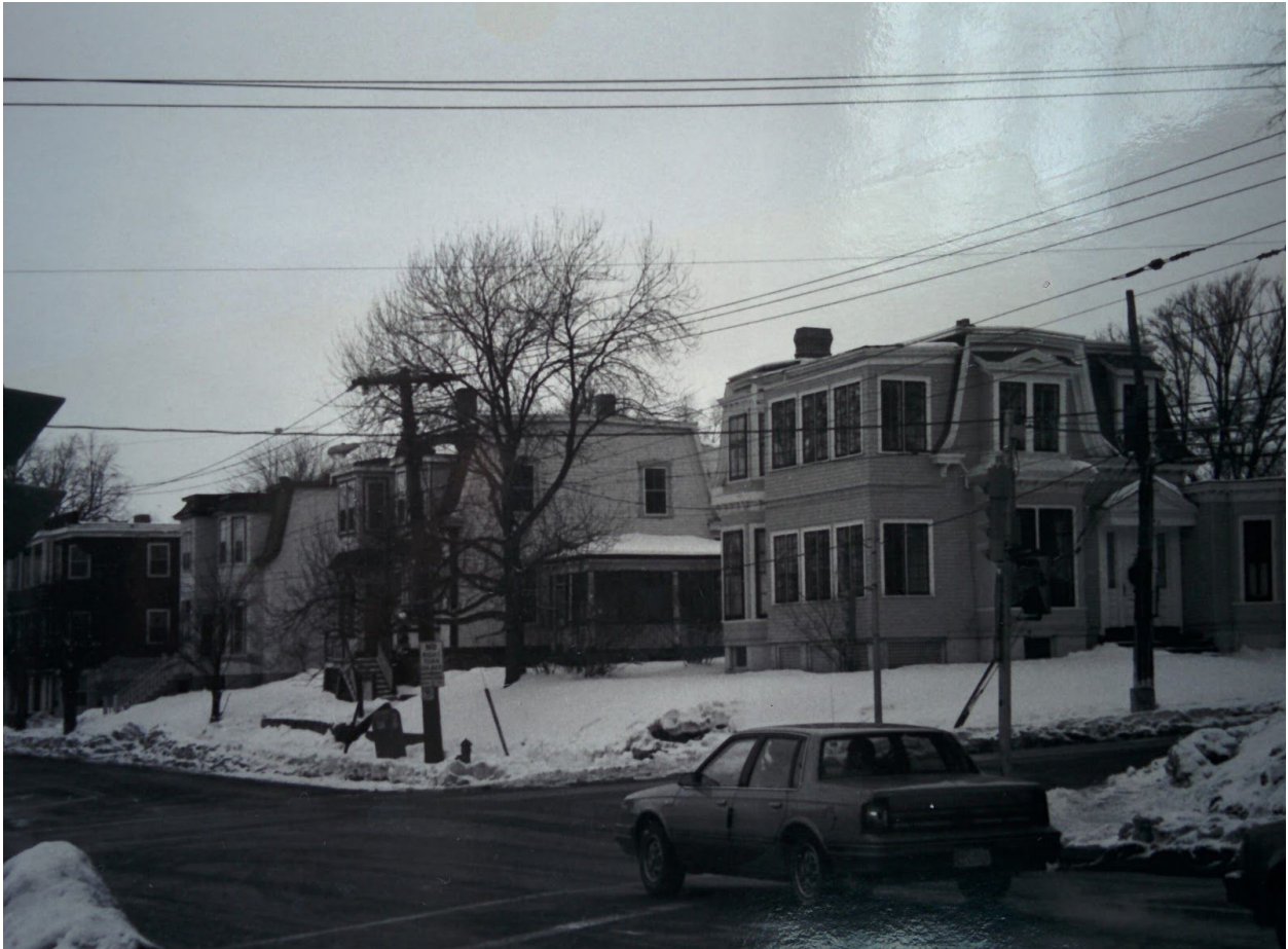
33-35 Pleasant Street visible in far left of photograph.
