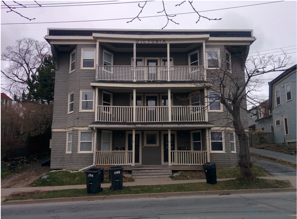
Site Visit - April 22, 2017
