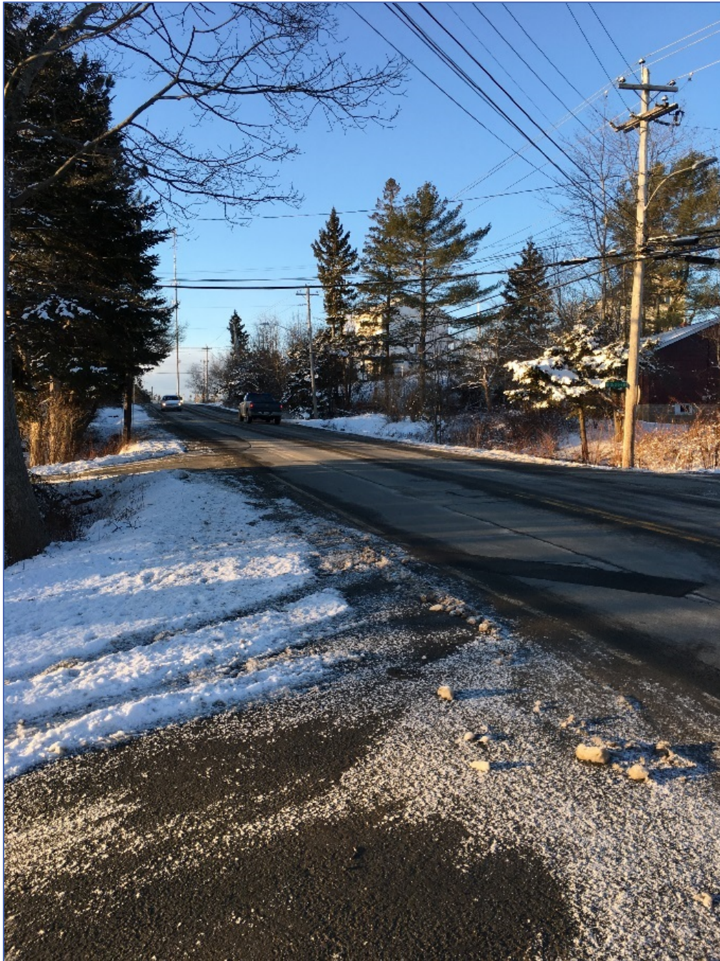
Figure 3 - Sight distance to the left at 429 Cobequid Road driveway
