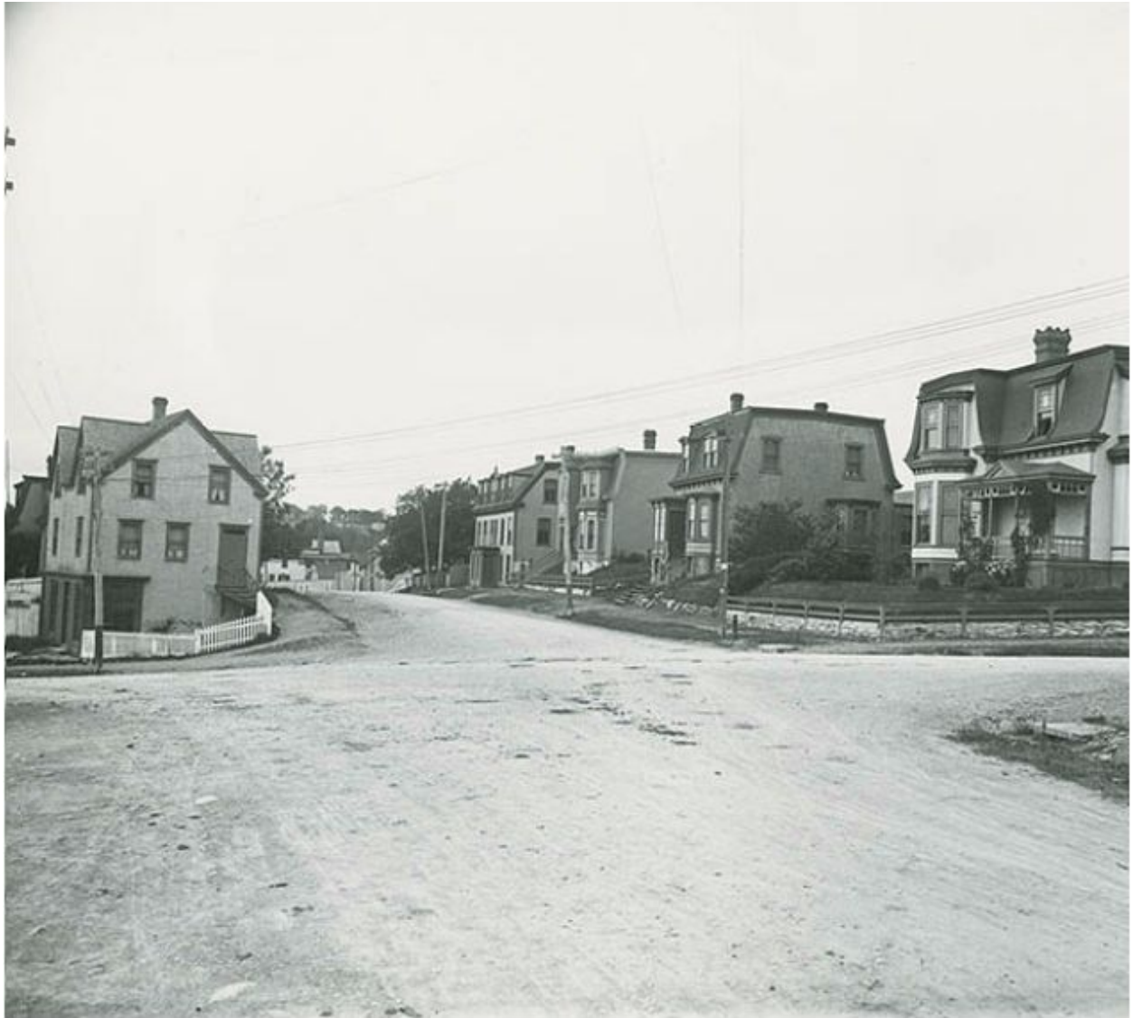
Original Photo, Five Corners looking down toward Pleasant Street. 33-35 Pleasant is the farthest house back.
