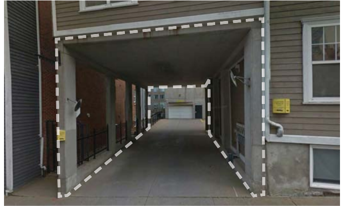
Figure 39. Existing Vehicle Portico Re-Instated & Improved
